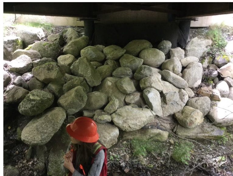
Left Bank Abutment when facing downstream
