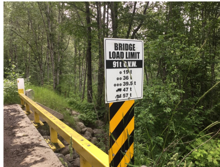
Load Rating Sign
