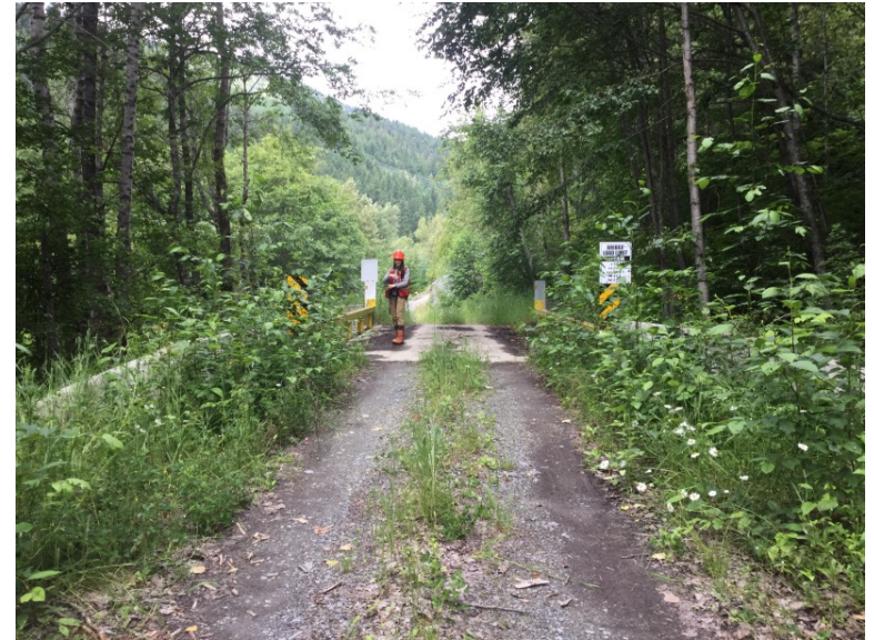
Right Bank Abutment when facing downstream
