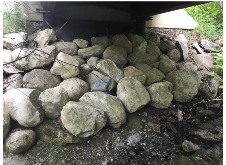
Right Bank Abutment when facing downstream
